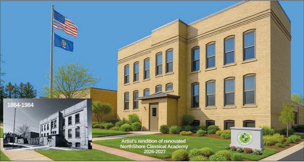
News Graphic file photo NorthShore Classical Academy will renovate the campus' two buildings — the first constructed in 1860 and the other in 1962.
